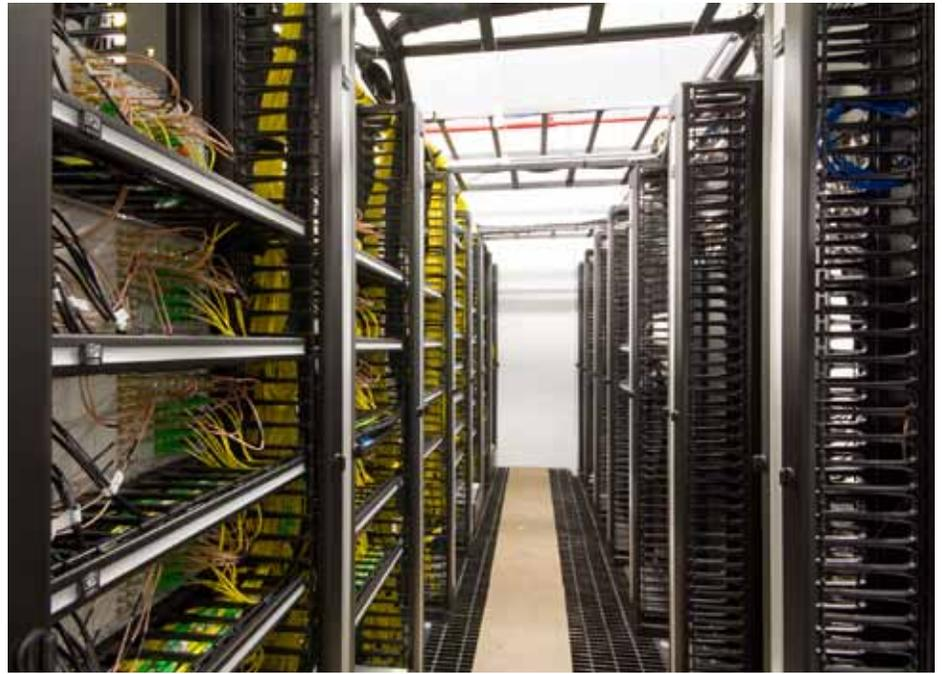
During a DAS deployment, wireless providers will need space for their head-end equipment (Source: Connectivity Wireless).
